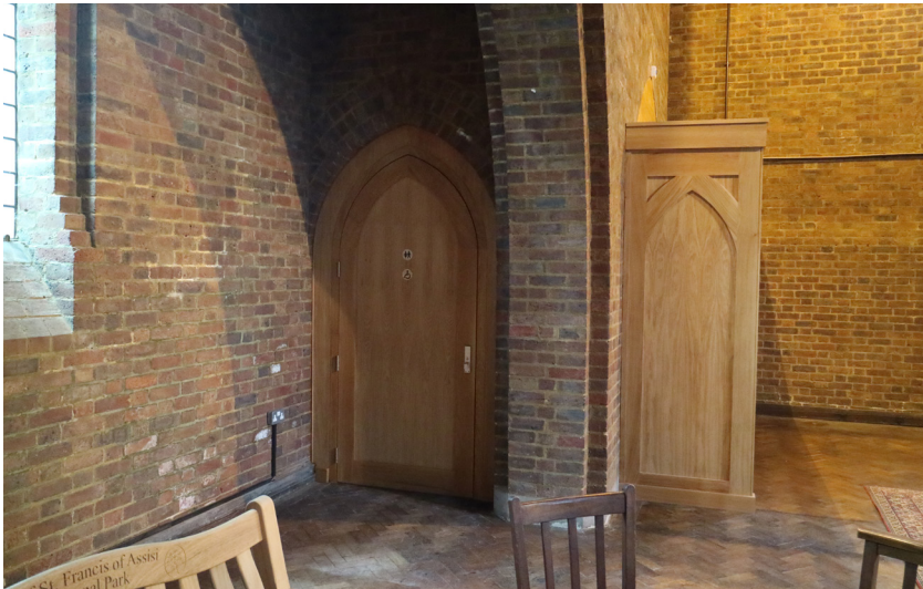
Infill to arcade with new oak door to WC and tea station cupboard on right
