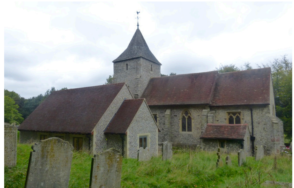
View of Cloisters extension from the south east
