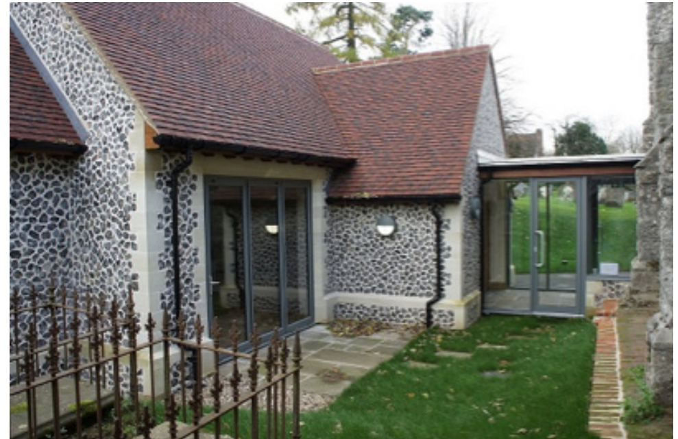
View of extension from the east showing the fully glazed link to the tower (photo by PCC)
