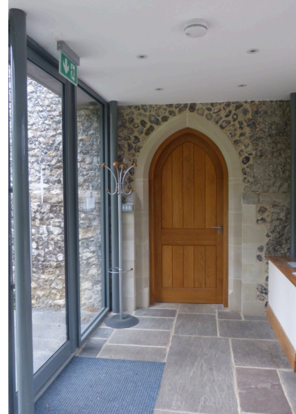
View inside link corridor looking towards the new tower door
