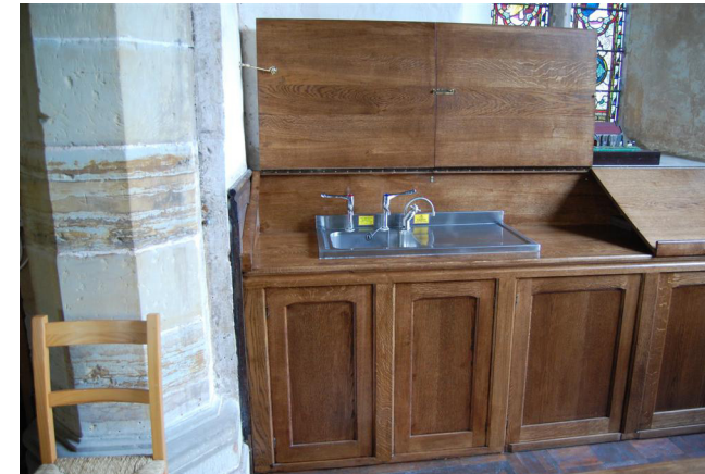
Tea station in partially open position to show sink unit
