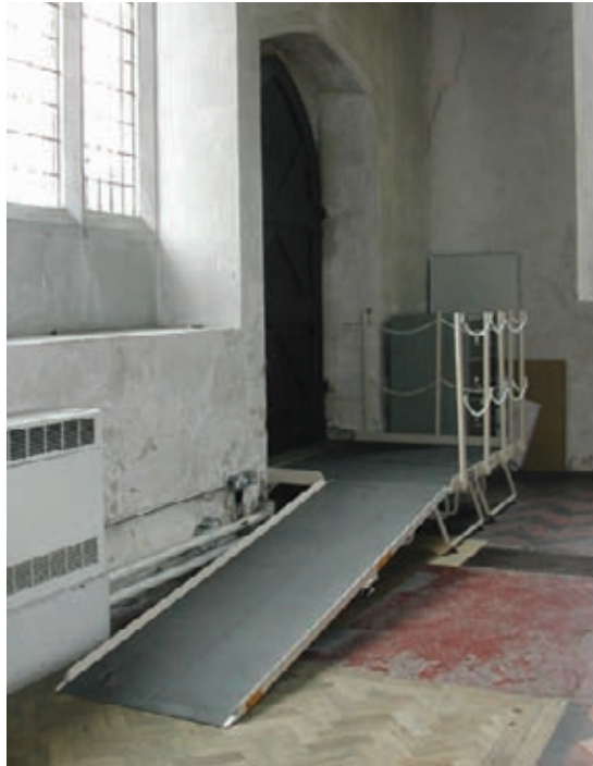
At St James' Church, Colchester, the level change at the north porch is more than a metre. A removable ramp at the south door provides access until a permanent solution is provided.
