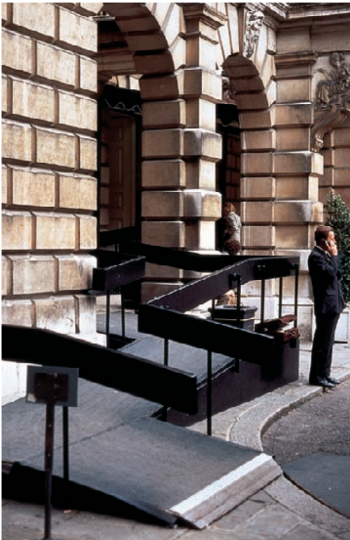
At the Royal Academy, Piccadilly, the permanent scheme (right) which replaced unsightly temporary ramps (left) involved the modification of the plinth to accommodate the raised courtyard levels. Picture to the left © Francis Ware
