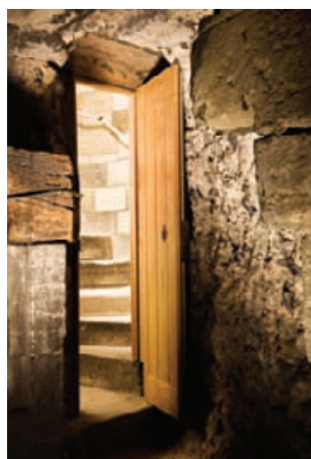
These fire doors at Winchester Cathedral were sensitively designed and custom made to fit a range of openings.
