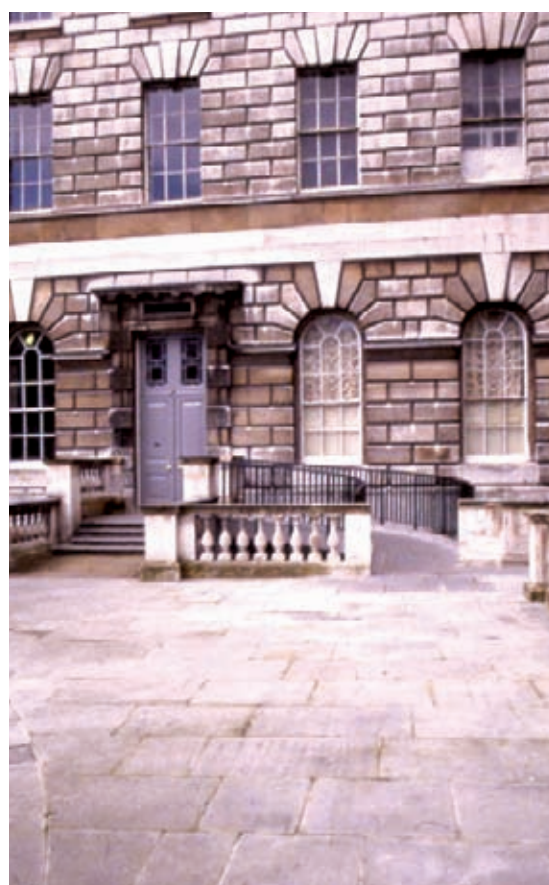
The stone balustrade has been cut through on one side of the entrance to the Seaman's Hall at Somerset House to provide ramped access.
