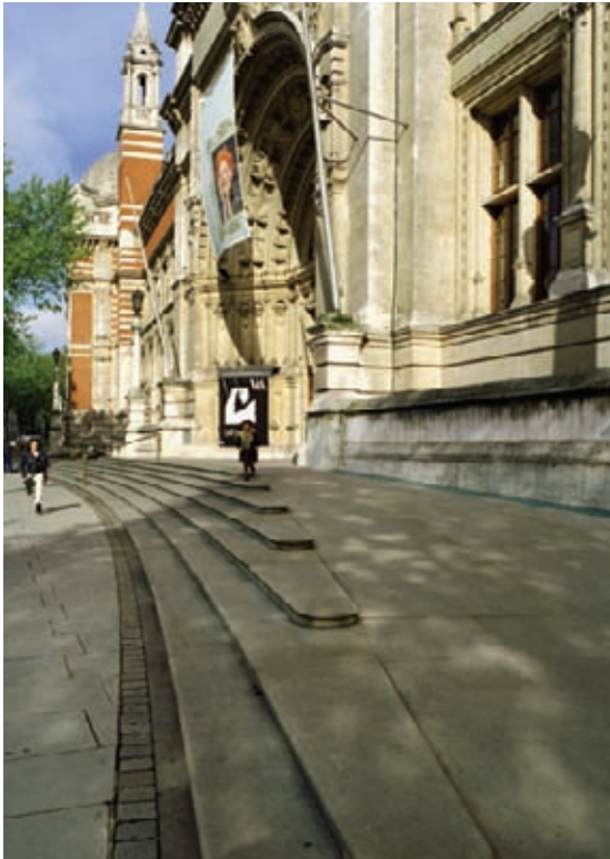
At the Victoria and Albert Museum in London long symmetrical shallow ramps have been combined with steps that complement the scale of the Cromwell Road frontage. There is one central handrail to the steps.
