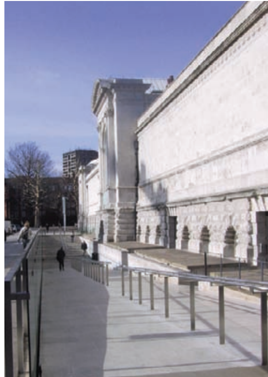
A new accessible entrance at Tate Britain has wide steps and ramps.
