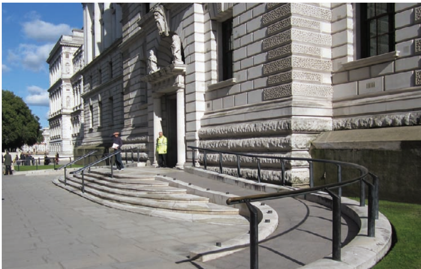
The refurbished entrance to the Treasury in Horse Guards Road has a symmetrical arrangement of ramp and steps. High-quality design complements the refurbishment of the historic elements.
