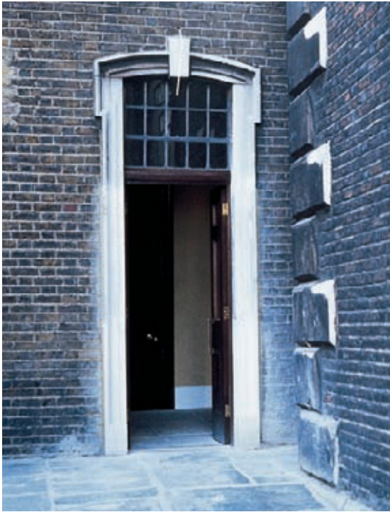
The Christopher Wren-designed church of St James sits between Piccadilly and Jermyn streets, which are at different levels. Level access has been achieved from Jermyn Street by altering a window to form a doorway, which is located in a 19th-century addition to the original body of the church and deemed less sensitive.
