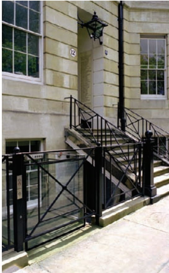
King's Bench Walk, Inner Temple, London. A short-rise platform lift is positioned behind railings where it descends to basement level and connects to the primary circulation routes.
