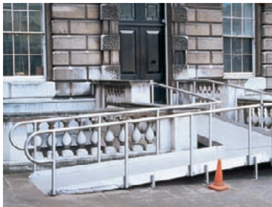
At St James' Church, Colchester, the level change at the north porch is more than a metre. A removable ramp at the south door provides access until a permanent solution is provided.
