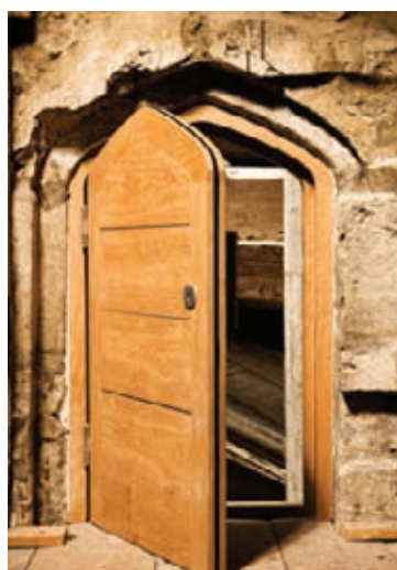
These fire doors at Winchester Cathedral were sensitively designed and custom made to fit a range of openings.
