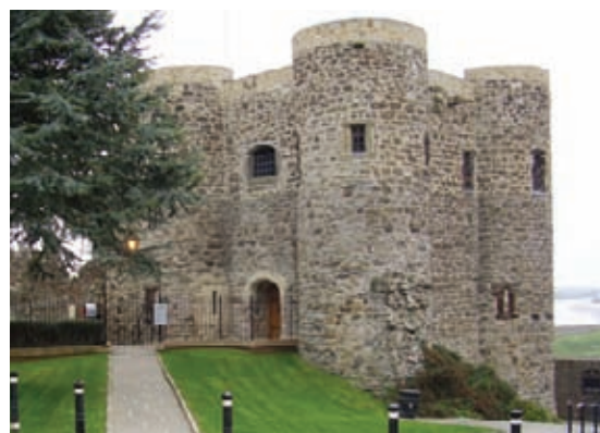
Access was improved at the scheduled Ypres Tower in Rye, East Sussex, by creating a gently sloping approach path across the lawn and reconstructing an original medieval doorway to give level access to the ground floor.
