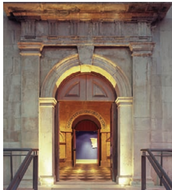
The once-derelict grade I listed church of St Luke in London has been converted into a community and music education centre for the London Symphony Orchestra. Access improvements to the entrance are sensitive to the architectural importance of the building.
