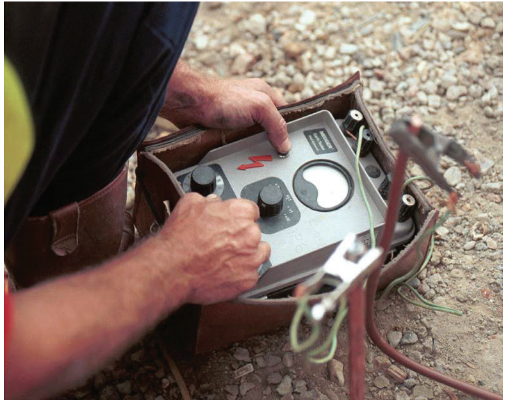
Figure 24: Engineer testing an installation.
