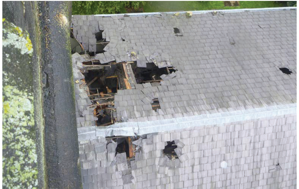
Figure 3, 4: Masonry debris from the tower fell through the roof of St Andrew's Church, Ramsbottom (Bury) causing extensive damage.
