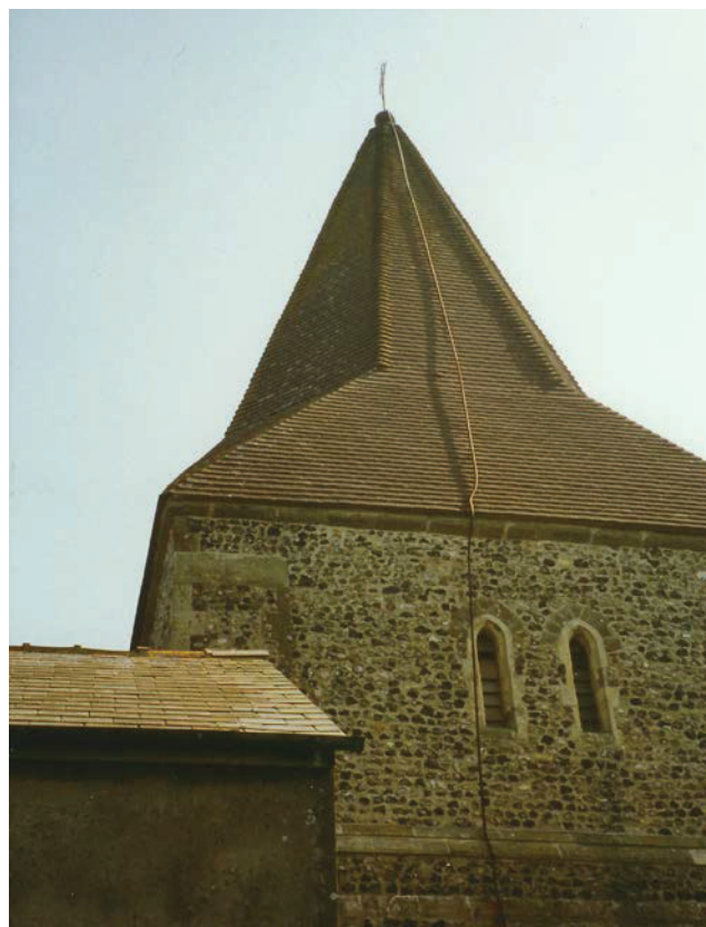
Figure 16: A very old and unusual iron conductor made of screwed sections at St Lawrence's Church, Hougham (Kent). Note the lack of support of the roof section.
